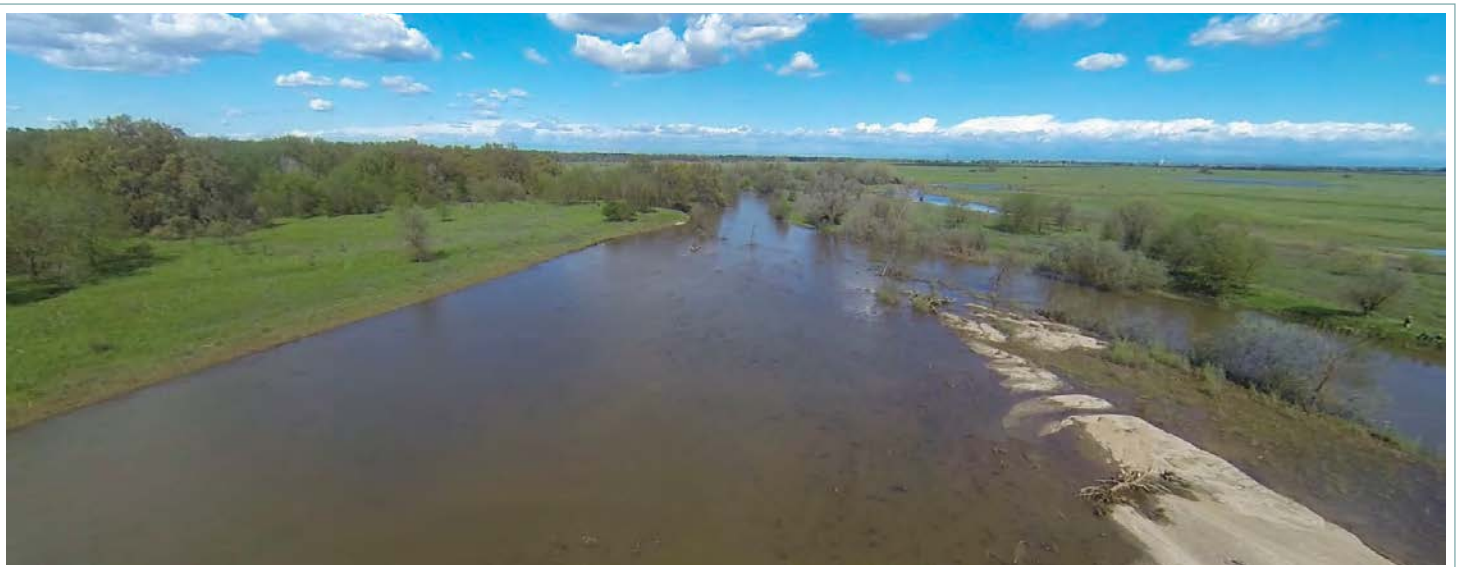
Cosumnes River levee breach. Photo: Lorenzo Booth/UC Merced
