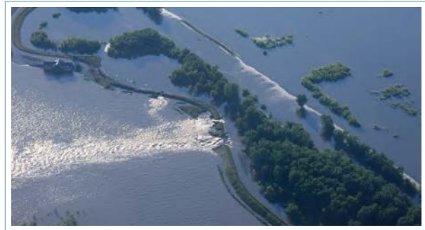
Mississippi River levee break. Photo: Jocelyn Augustino/FEMA
