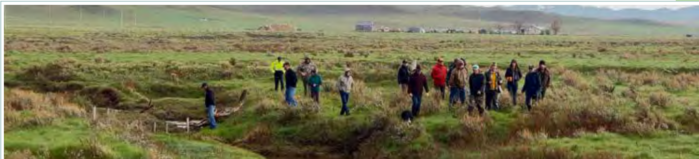
BDAs installed at Winifred project site in partnership with Bureau of Land Management, Montana Wildlife Federation, National Wild Turkey Federation, National Fish and Wildlife Foundation, and private landowners. Credit: Bureau of Land Management
