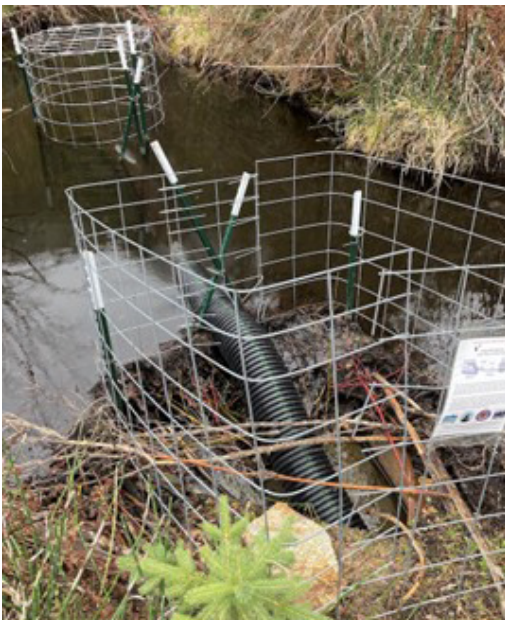
Figure 26: An example fence and pipe device installation. Device designs are site-specific and using the basic design principles, can be adapted for a variety of different waterways by a trained professional. Photo Credit: Elissa Chott.
